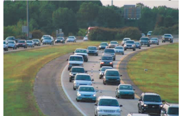
Figure 6.3.1: I-40 near US 1 Interchange
