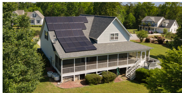
Solarize the Triangle Installation
