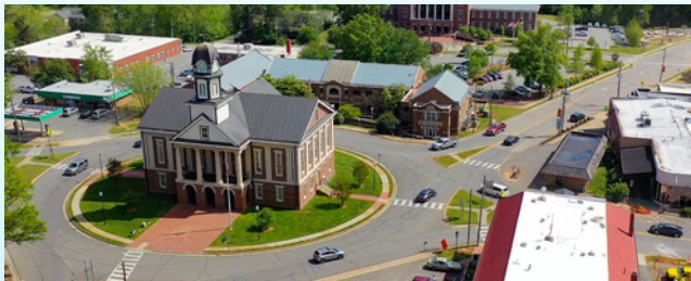
Chatham County Courthouse, located in Pittsboro
